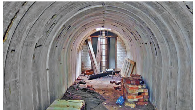
Looking towards the escape ladder and chemical toilets in one of the shelters. Photo Chris Rayner
